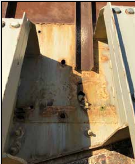
Examples of damage and wear due to constant contact of rock and sand.
